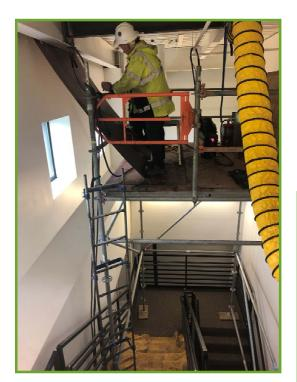
Special inspection of the welding the Davit Arm support to the building structure
