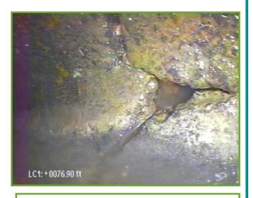
Crack on side of sewer pipe
