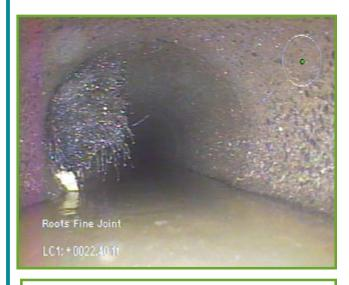
Root intrusion into sewer pipe
