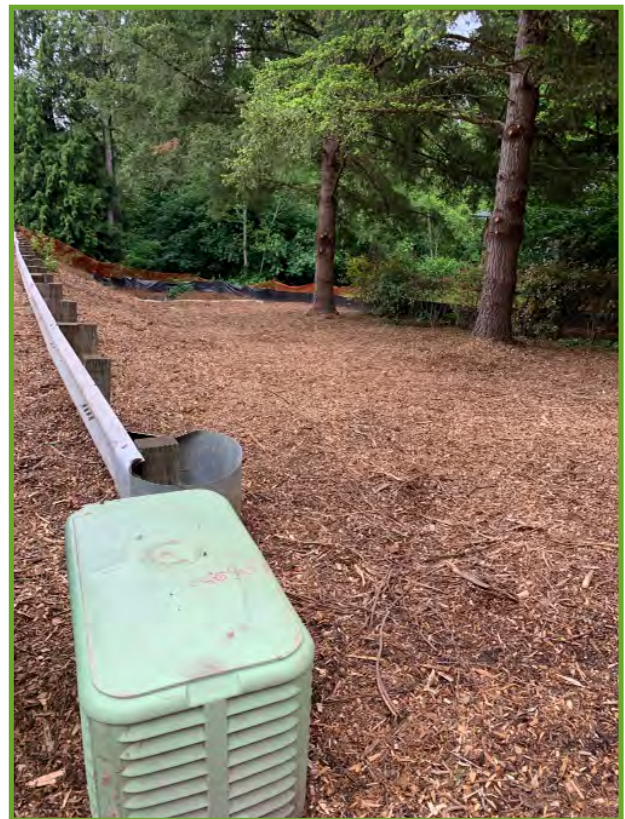
Looking west towards Boeckman Creek with the temporary erosion control measures in place.
