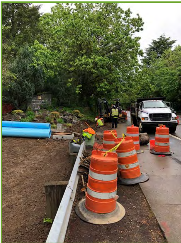
Project work site along Wilsonville Road.
