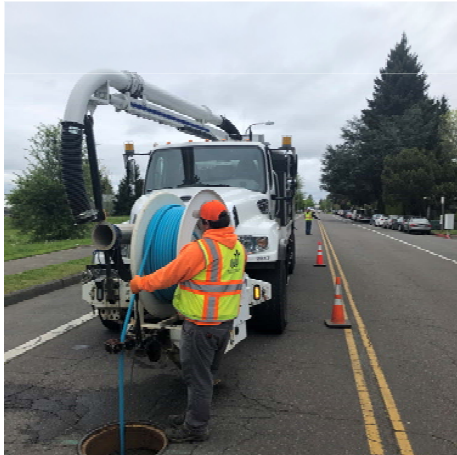
Cleaning sewer main
