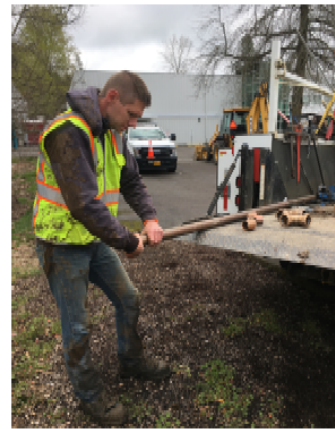
Preparing new copper pipe
