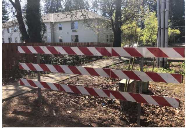
Replacement barricade with steel posts
