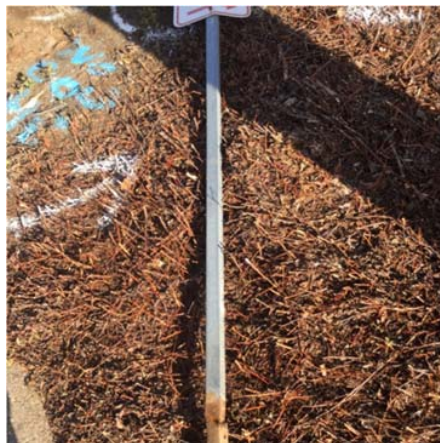
Downed “No Parking” sign needing to be replaced
