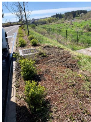
Restoration of sink hole area
