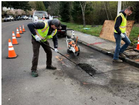
Removing asphalt pavement
