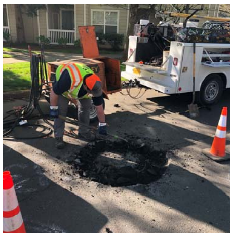
Preparing foundation for casing ring installation
