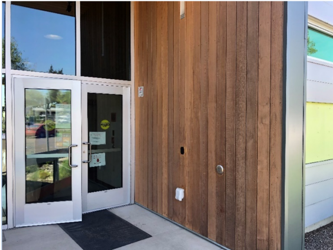
Photo 16: SMART Facility Entrance
