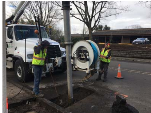
Excavating hole with vacuum truck
