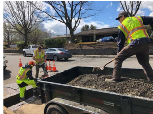
Backfilling excavation
