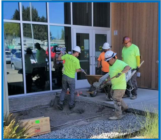
Parking lot construction and front deck addition
