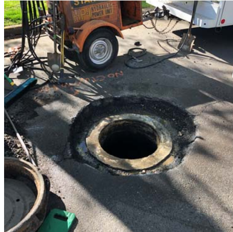
Removing casing ring foundation
