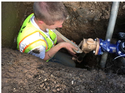
Tightening pipe fittings
