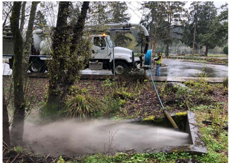
High water pressure was used to clear the blockage
