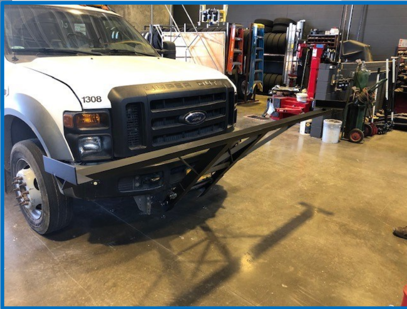
Completed framework in place, awaiting final plumbing of hoses and spray nozzles
