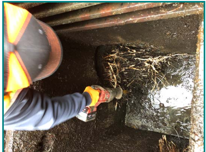
Randy Burnham cutting root out of a catch basin with saw
