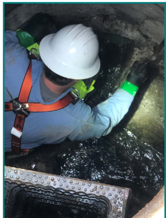
Kyle Bean in a Sewer Manhole
