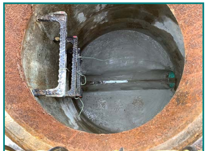
Repaired Manhole Channel
