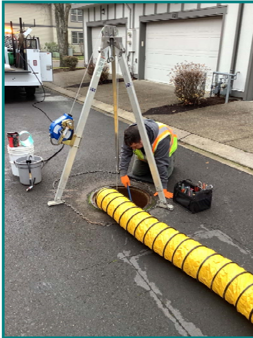
Chad Whiting — Venting Manhole for Clean Air
