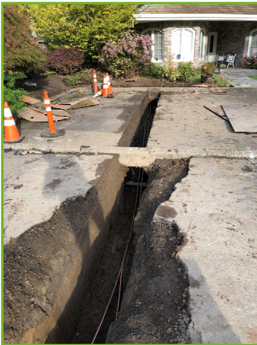
Trench for new water line
