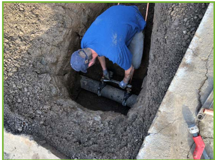
Water Technician Sam Kinnaman installing service lines
