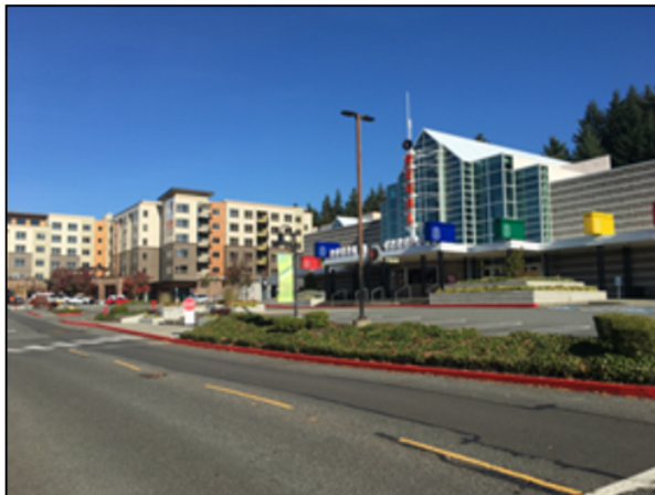
Crossroads Bellevue is transitioning from a strip commercial center, adding multi-family housing, office and additional retail opportunities.
