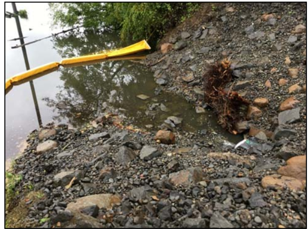
Completed Belnap Court Outfall.
