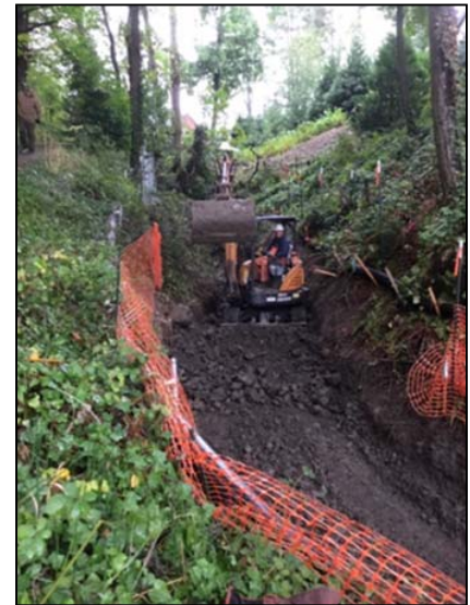
Morey Court Channel Construction.
