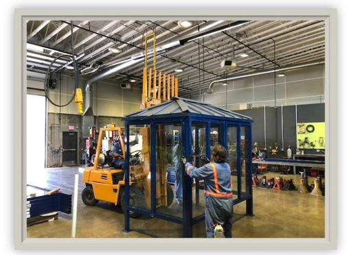
These shelters are assembled in the Fleet shop, and Public Works handles the on-site installation.
