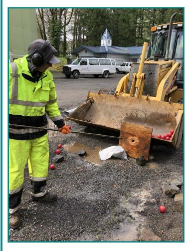
Paul Walker demonstrates the power of the high pressure hydro excavation wand by cutting through a piece of ply-wood.
