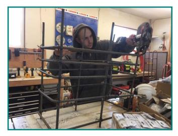
Back at the maintenance shop, crew members cut rebar and built the reinforcement cage to be installed during the concrete pour of the footing.
