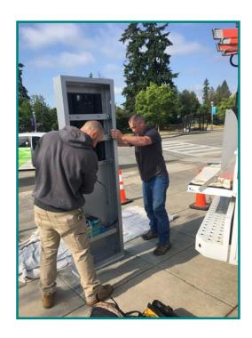
Next the solar panel had to be attached to the top of the reader board, wires inside of the unit were plugged into the appropriate terminals and the back panel was fastened to the unit with tamper proof screws. Finally, crew members called the vendor to confirm that the reader board was powered up and working properly.
