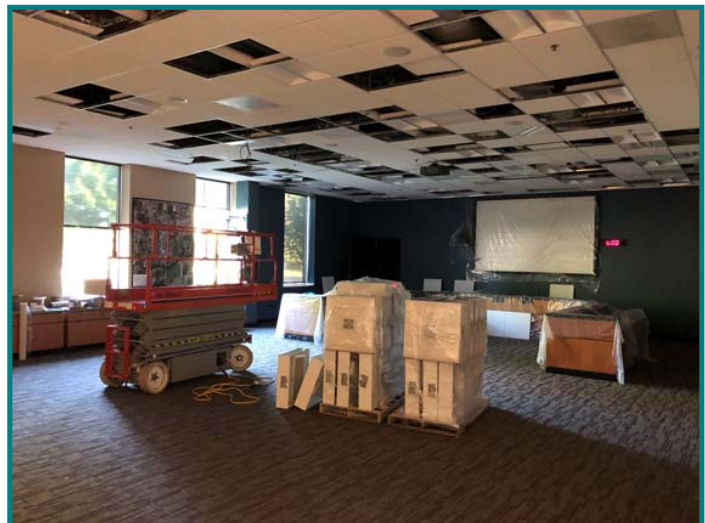
During Project Construction - Council Chambers
