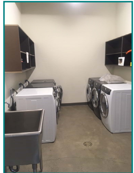
Dedicated washers and dryers for soiled or contaminated uniform items.
