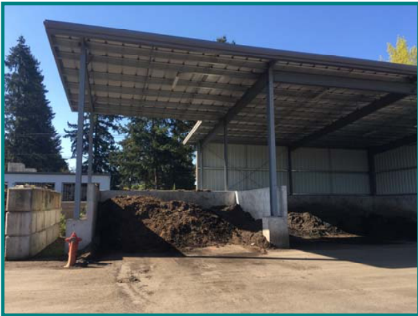
Decant facility for Vector & catch basin materials.
