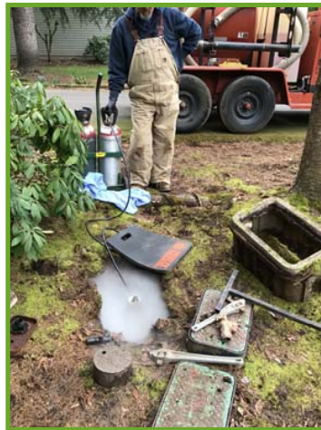
Water Technician Sam Kinnaman installs the freeze kit cuff around the service line to be frozen.
