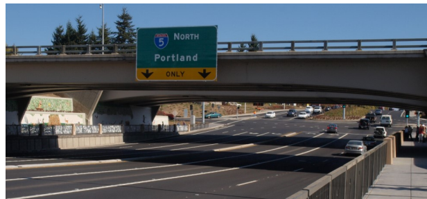
Looking east to the I-5/Wilsonville Road interchange.
