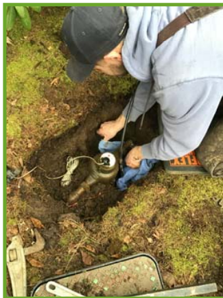
Water Technician Sam Kinnaman installs the freeze kit cuff around the service line to be frozen.
