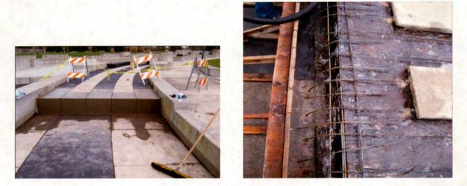
Once the repair was finished, the City's contractor, Aldercrest Construction was able to finish the staining project. The staining of the concrete was an attempt to restore the black color of the concrete so that the original design of the water feature would be reestablished. The project included cleaning of the concrete, application of two coats of stain and one coat of sealer. Notice the difference in contrast in the photos below.
