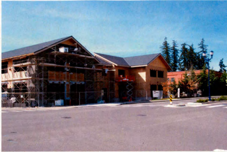
Boone Building near Old Town Square
