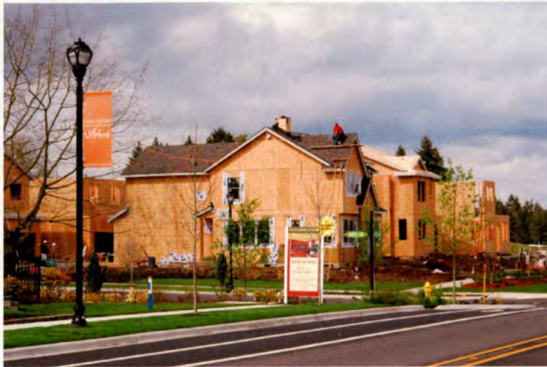
Polygon Homes construction at Villebois
