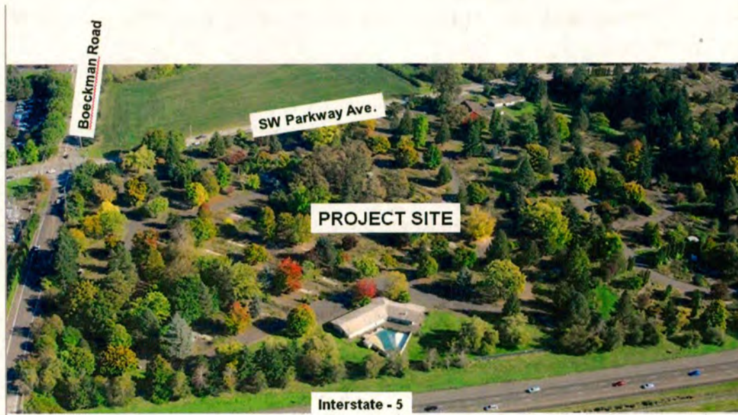
BRECHLEY ESTATES - NORTH SITE LOOKING EAST
