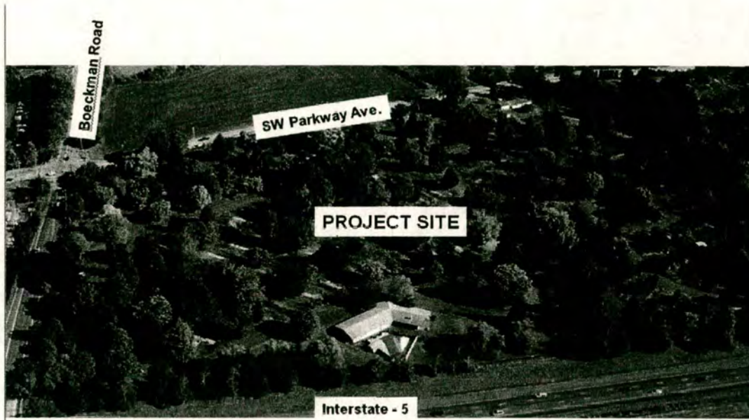
BRECHLEY ESTATES - NORTH SITE LOOKING EAST
