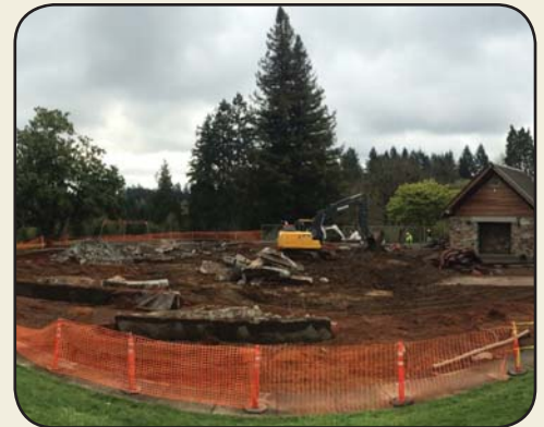
Began demolition of Murase Plaza play equipment
