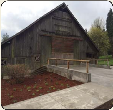
Completed Stein-Boozier Barn gathering area concrete and landscaping
