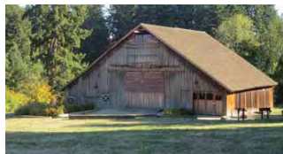
Stein-Boozler Barn - Access Improvements
