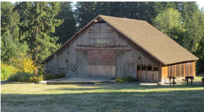
Stein-Boozier Barn - Access Improvements
