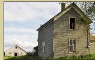
The Bill Bischof house and barn, now demolished, were south of the Boeckman crossing in the Villebois neighborhood.
