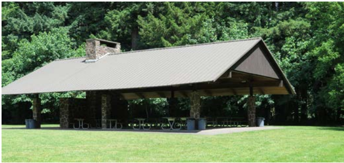
Existing River Shelter
