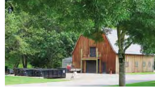
Future Picnic Shelter with Restroom
