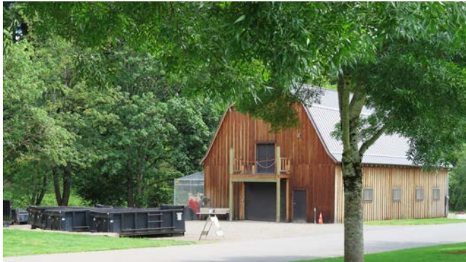
Future Picnic Shelter with Restroom
