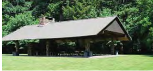
Existing River Shelter
