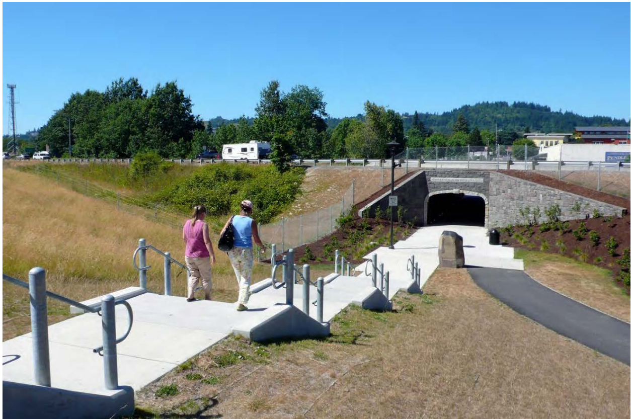
After: South end of SR 14 Pedestrian Tunnel, with stairs and ADA-accessible path connecting to fitness trail along the top of the Columbia River dike
