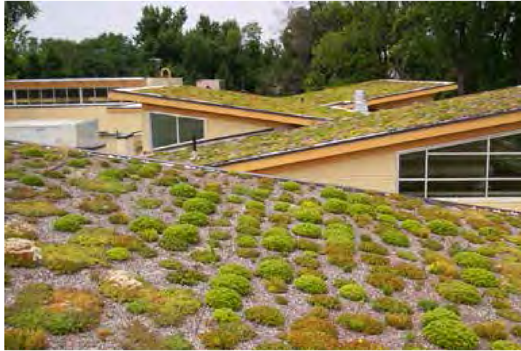
Green Roof (Reduces roof runoff and improves building insulation)
