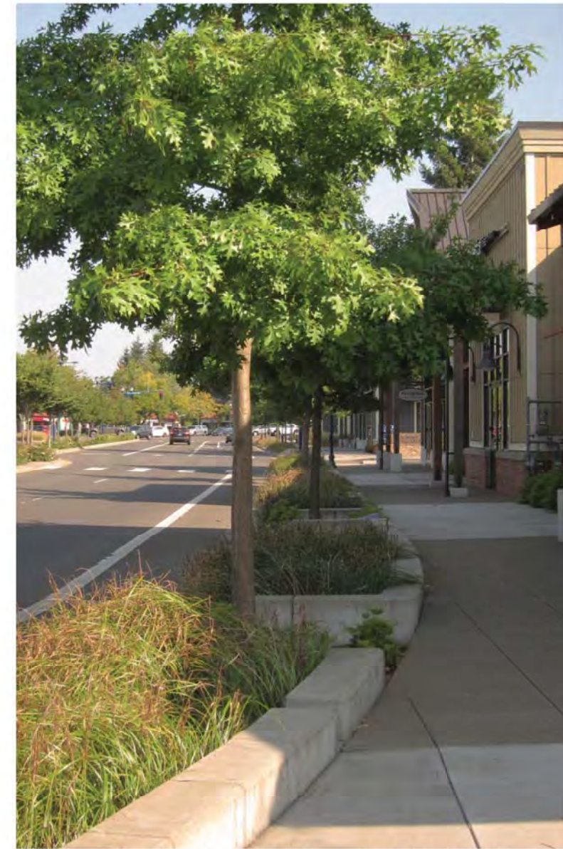
Stormwater treatment integrated into Main Street
