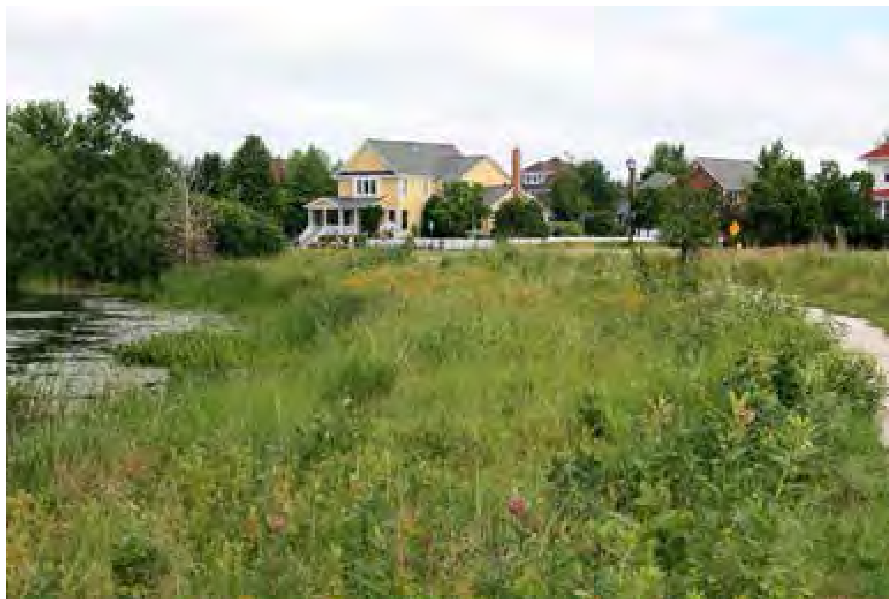
Retention Pond (Holds rainwater in wetland environment)
