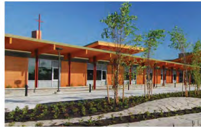
Civic Buildings on a small public plaza
