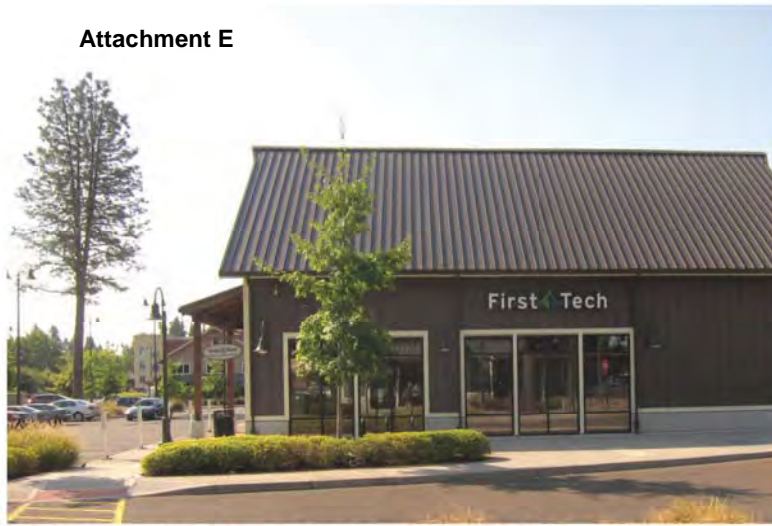
Neighborhood-scale commercial building
