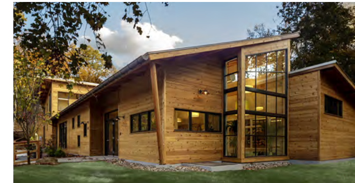
Small daycare and community use building
