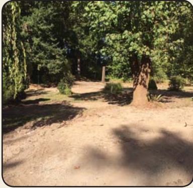
Completed clean up of the Duckworth Property adjacent to Boones Ferry Park
