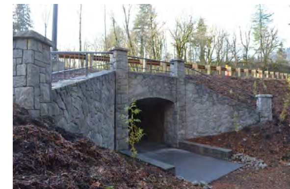
UNDERCROSSING EXAMPLE 2: SR-14 Tunnel in Skamania County, WA
