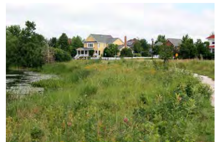
Retention Pond (Holds rainwater in wetland environment)
