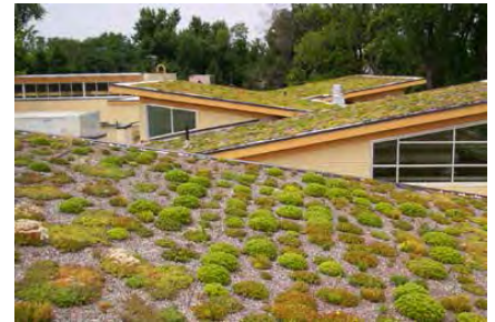
Green Roof (Reduces roof runoff and improves building insulation)
