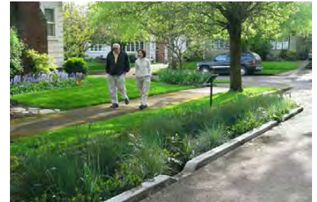
Stormwater Bioswale (Natural detention and filtration of on-street rainwater)
