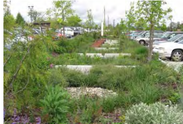
Parking Lot Rain Garden (Natural detention and filtration of parking lot rainwater)
