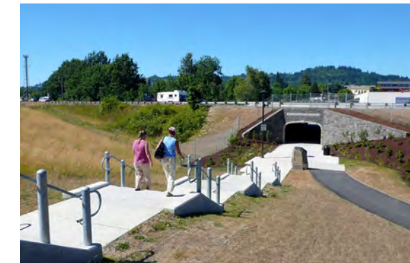
After: South end of SR 14 Pedestrian Tunnel, with stairs and ADA-accessible path connecting to fitness trail along the top of the Columbia River dike
