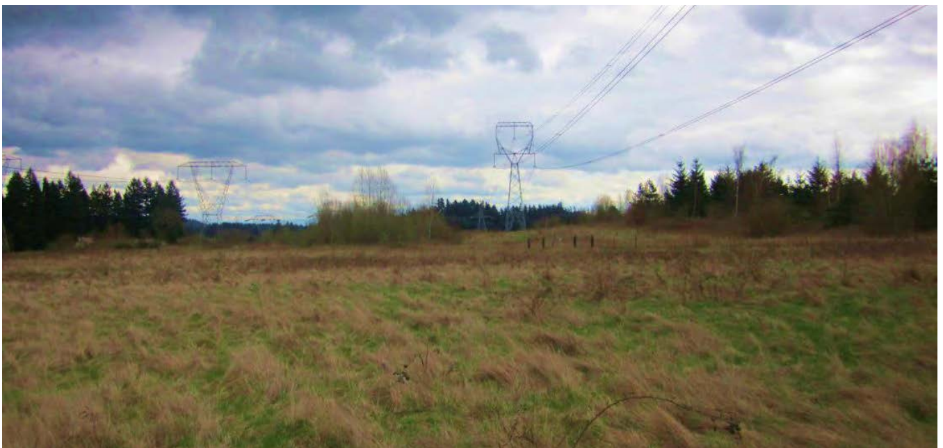
Figure 28. Existing BPA Corridor
