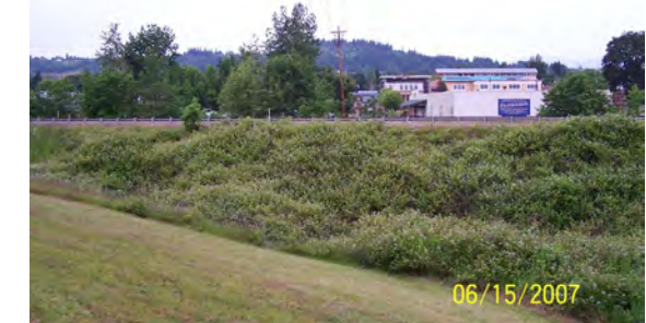
Before: South side of SR 14
