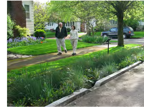
Stormwater Bioswale (Natural detention and filtration of on-street rainwater)
