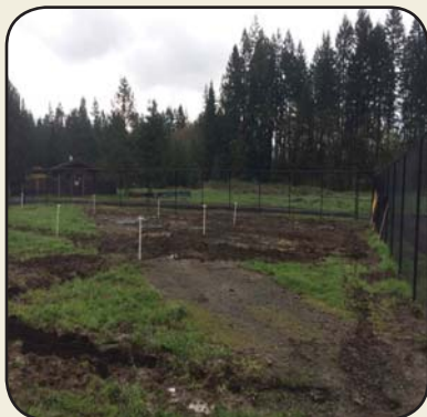
Completed fence and irrigation install at Community Garden
