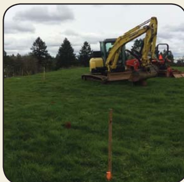
Began Murase Plaza Regrade and Terracing
