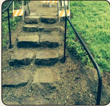
Completed steps and installed handrail at Stein Boozier Barn
