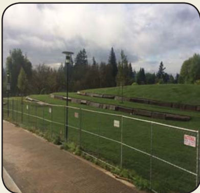
Completed Murase Plaza terracing project
