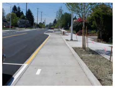
One-Way Cycle Track on Cully Boulevard in Northeast Portland. Cycle tracks are typically protected from motor vehicle traffic by parked cars, raised curbs, or other physical buffers.
