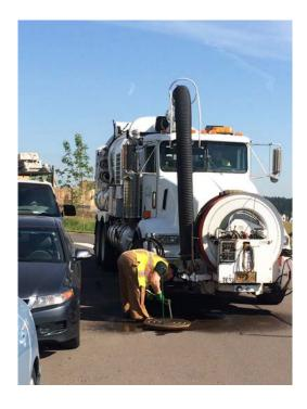
The Collections crew also helps other other crews by hydroexcavating to pothole for utilities and excavate water leaks. Vactor Operators Mark Folz and Paul Havens help the Water crew excavate a water leak on Orchard Drive which was obviously caused by tree roots.
