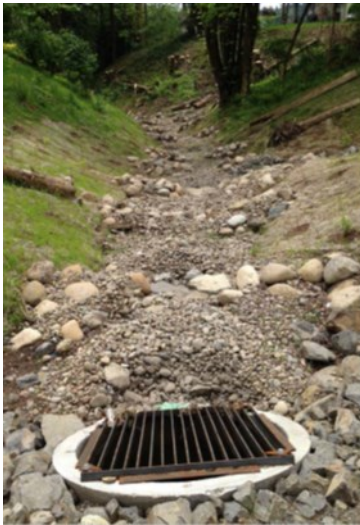
Morey's Landing channel and outfall (2014)
