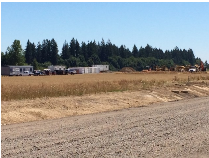
Meridian Creek Middle School Site
