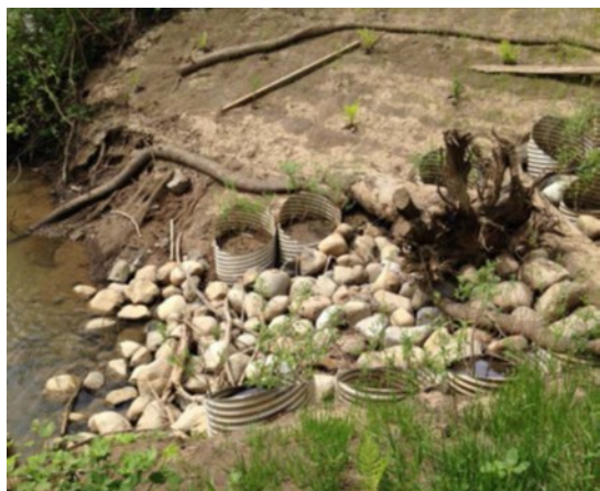
Rivergreen channel and outfall (2014)
