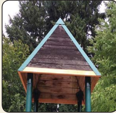
Replaced Worn Roof Pieces at Town Center Park Playground
