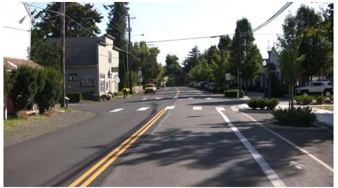
Intersection of Boones Ferry Road and 5 th Street. Older buildings on left sit on or over the edge of right-of-way.
