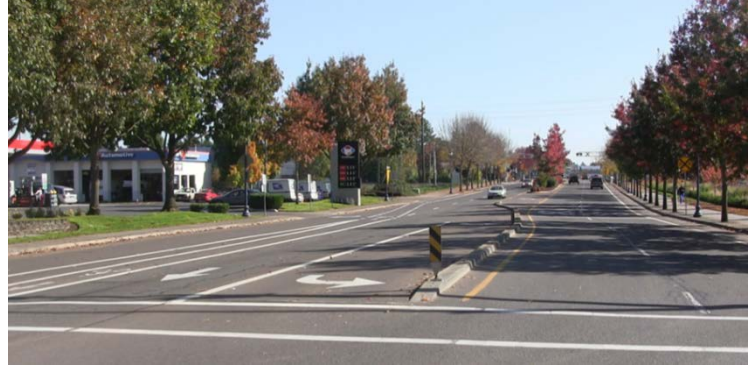
Bicycle lane on Wilsonville Road
