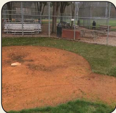
Stripped, re-graded, and re-sodded behind home plate on fields 3 and 4 to improve surface drainage and batters box conditions
