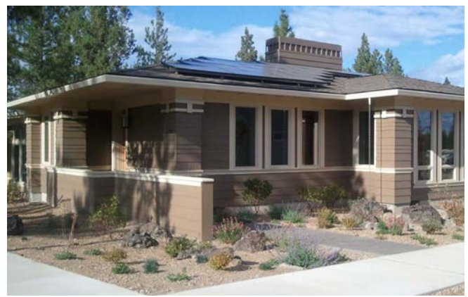
High quality construction, detailing, and diverse architectural styles make a neighborhood more attractive.
