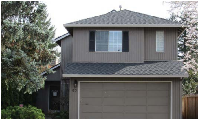
Houses where windows and doors are hidden from the street detract from the perceived safety of the neighborhood, because no one is aware of what happens in the street.
