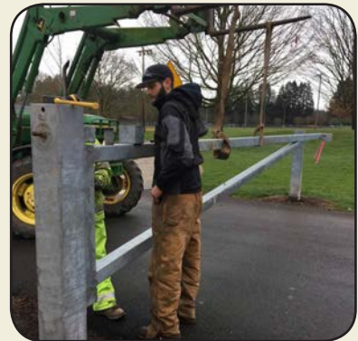
Replaced damaged gate at Memorial Park
