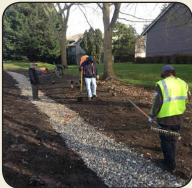
Completed planting at the Parkway Stormwater Project
