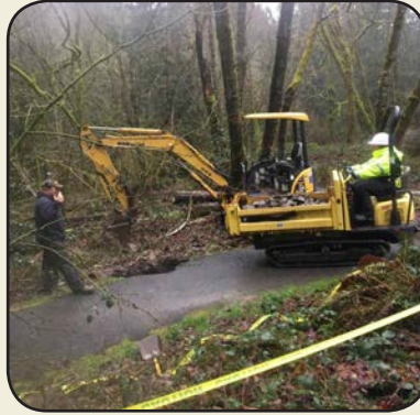
Repaired Boeckman Creek Trail Sinkhole
