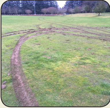
Began repair of vandalism at Memorial Park soccer fields
