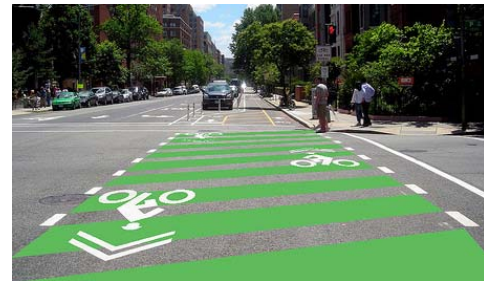
Cycle Track Crossing
