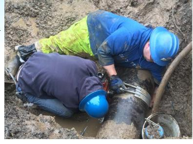
Water Distribution Technician Jerry Anderson puts together rigid copper pipe and fittings while Sam and Rick position the line prior to supporting it and backfilling.
