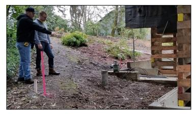
Pascoe is seen verifying the installation of a survey monument that is placed by a licensed surveyor. This monument is cast in concrete and indicates the floodplain elevation level for a 100-year event.
