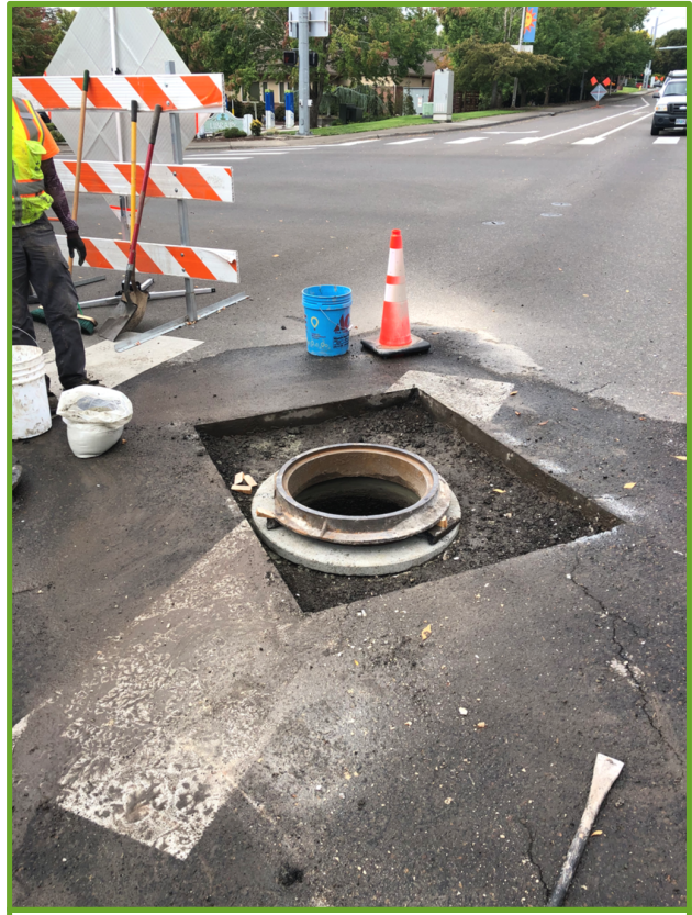
Excavated stormwater manhole
