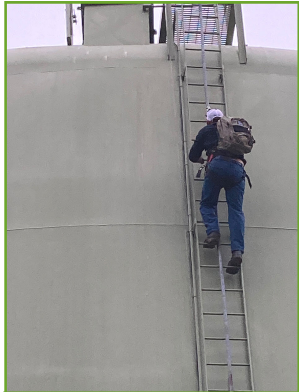
Contractor performing an inspection
