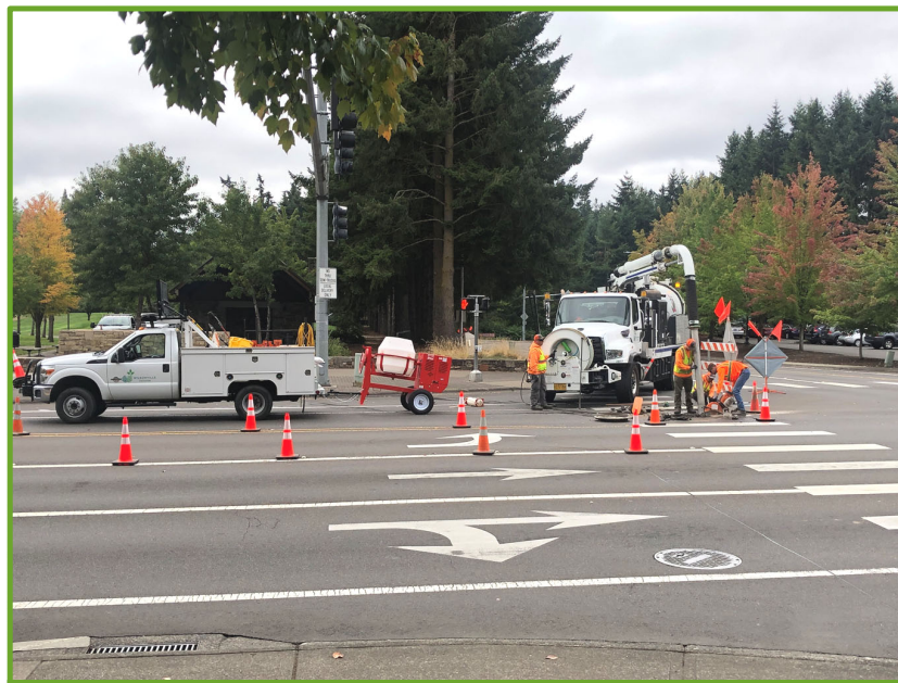
Traffic control for the work site
