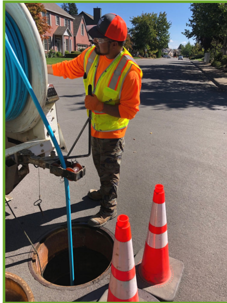
David cleaning a sewer main
