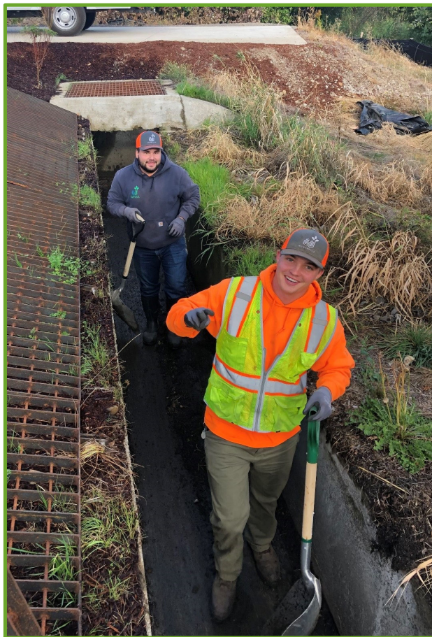
Roman and Konnen cleaning out level spreader
