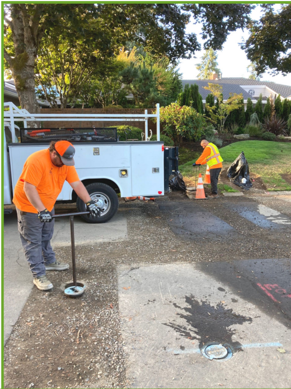
Chad & David shutting off a water main
