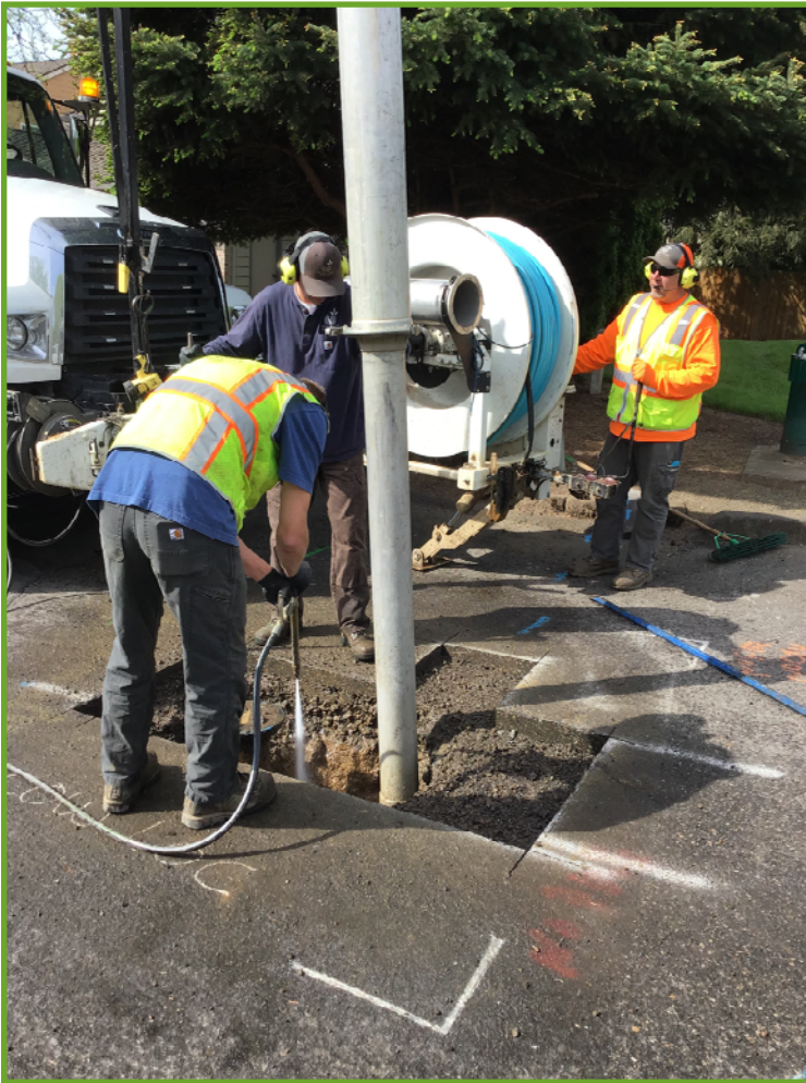
Using the vacuum truck to excavate trench
