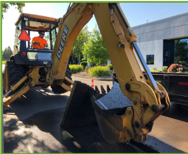
Removing Asphalt
