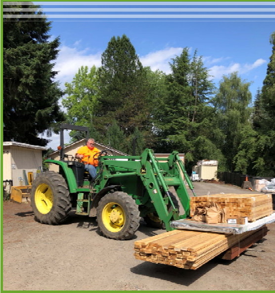
Facility Maintenance Specialist Robert Todd, loads the lumber for the deck railings on the trailer for transport
