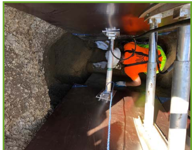
Working in the trench
