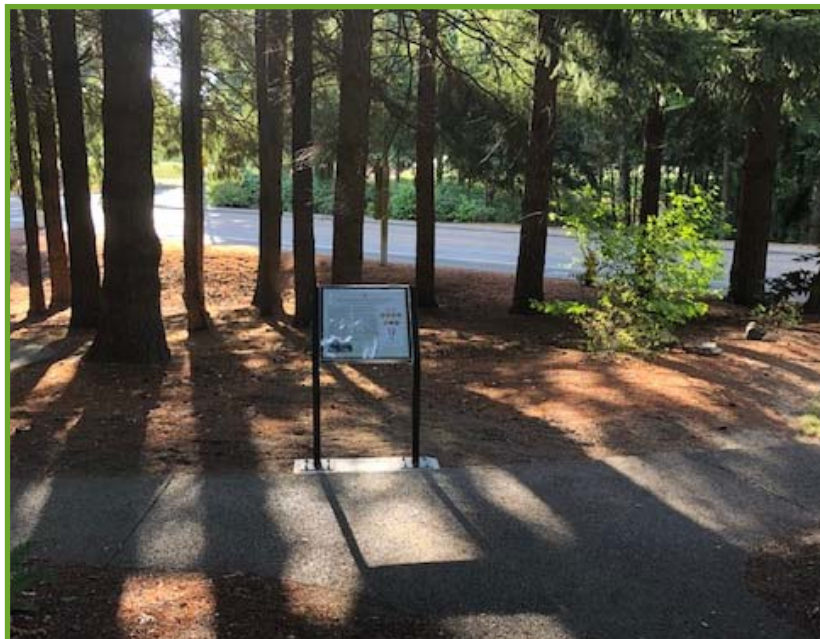
New sign sits upon a the new footing
