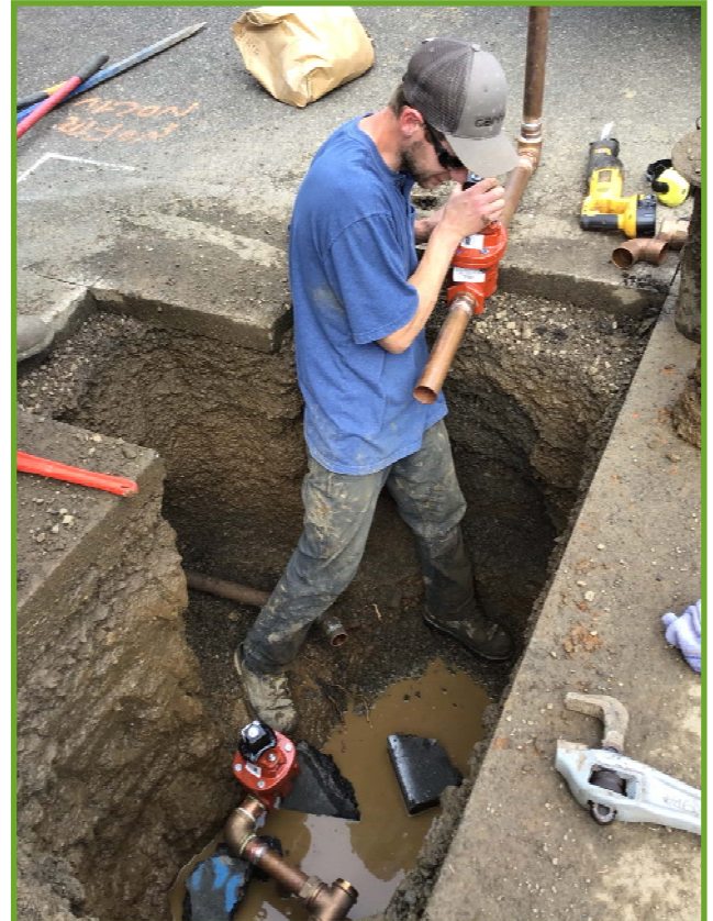
Installation of blow off valve
