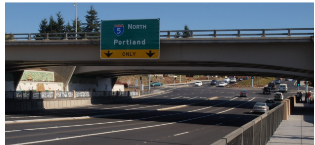
Looking east to the I-5/Wilsonville Road interchange.
