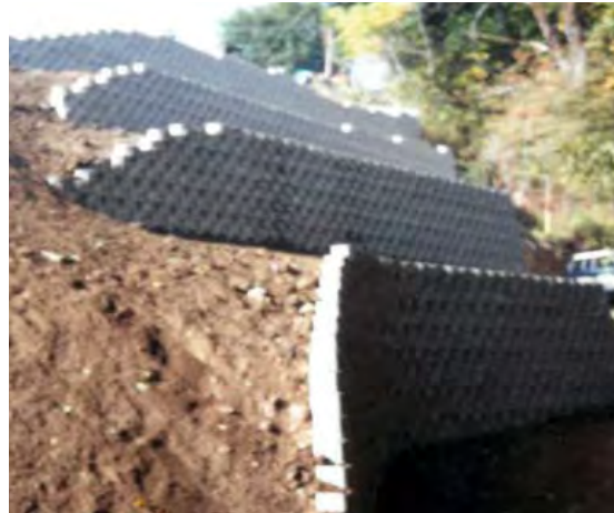
Access road and retaining wall in the Portland metro area
