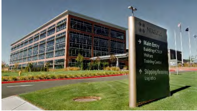
Figure 31 Lam Research Facility, Tualatin. Photo credit: Tualatin Chamber.
