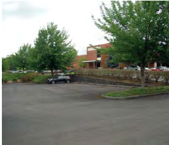
Parking lot retaining wall at Legacy Medical Office Building, Tualatin
