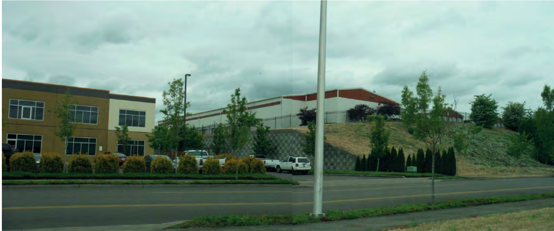
Office and commercial building near SW 124th Ave and SW Leveton Dr, Tualatin with retaining wall between properties
