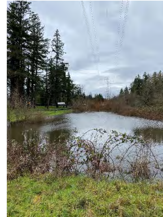
Ponding north of Day Road (Jan 2022)
