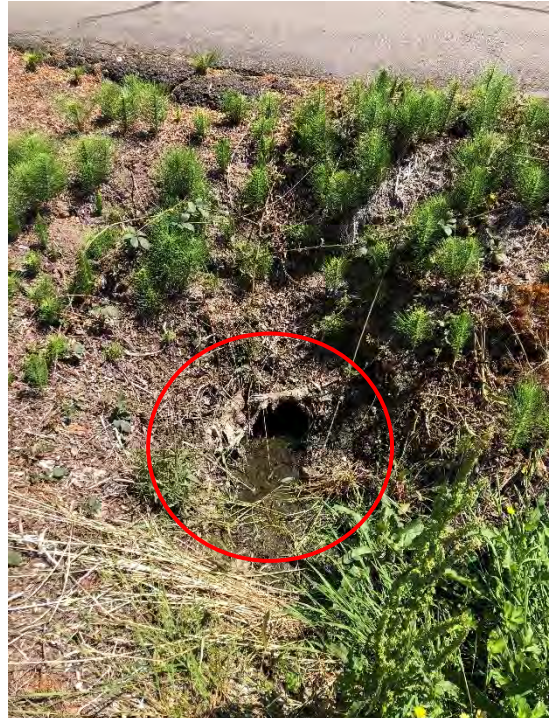
Culvert inlet under Rose Lane (May 2023)
