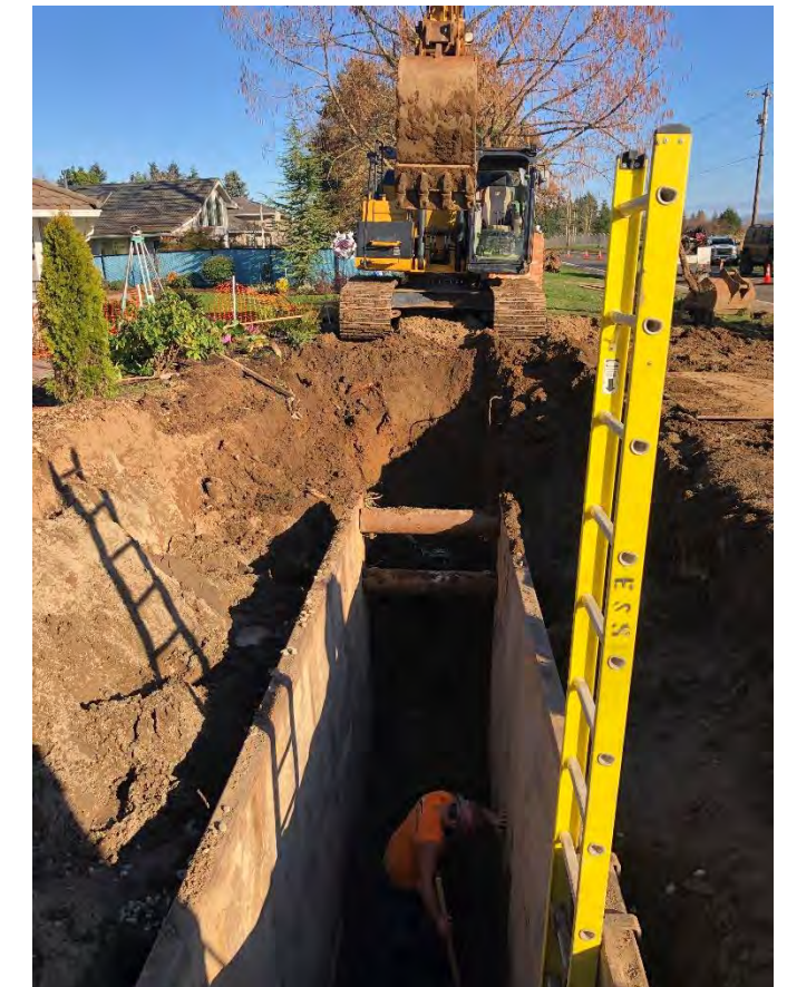
Temporary construction work on sinkhole
