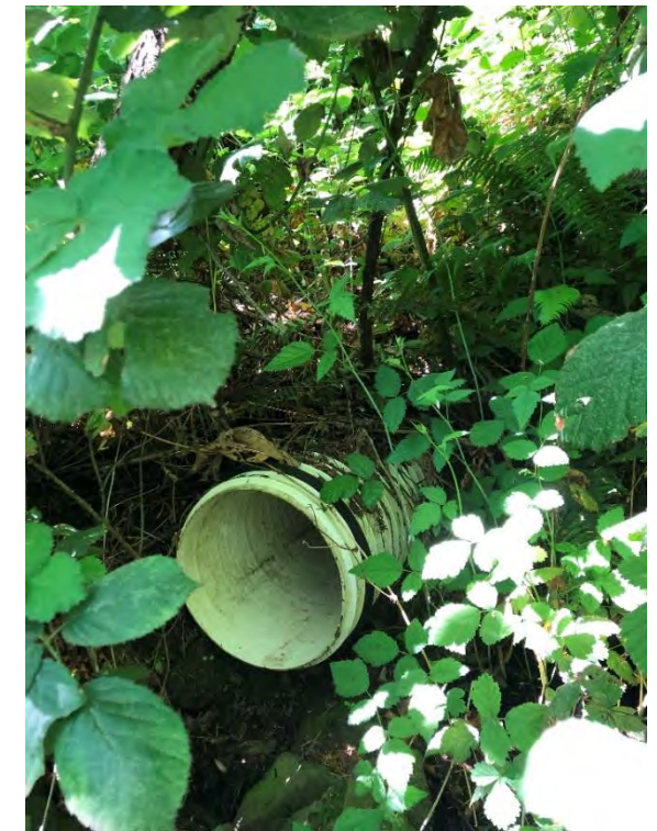
City-owned outfall pipe (May 2023)
