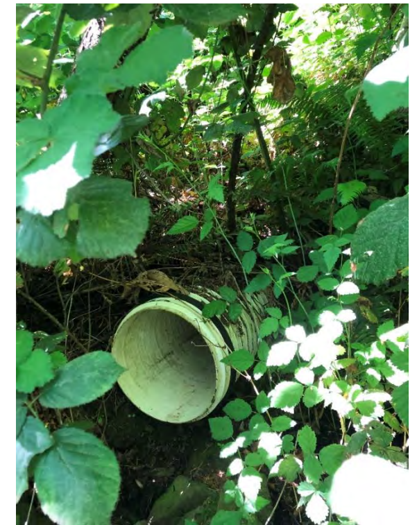
City-owned outfall pipe (May 2023)
