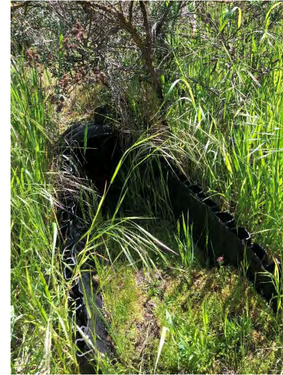
Garden Acres Pond Existing Inflow Pipe (May 2023)
