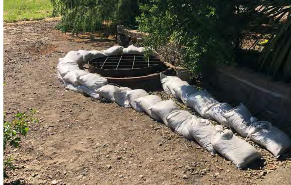
Existing Bubbler Structure (May 2023)
