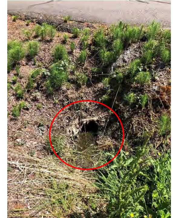
Culvert inlet under Rose Lane (May 2023)
