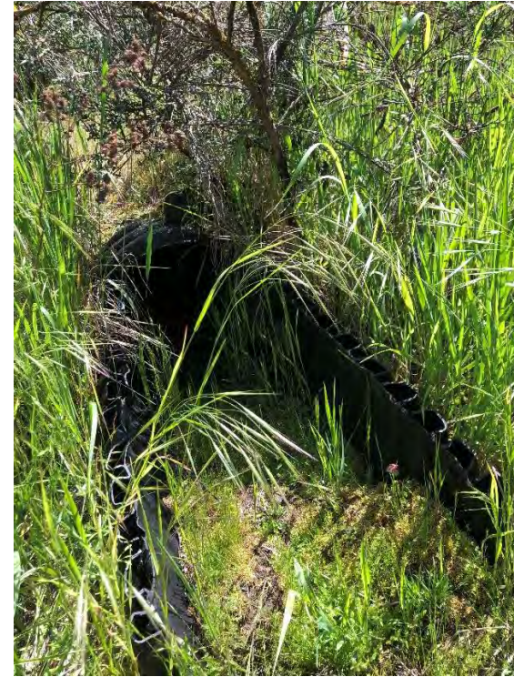
Garden Acres Pond Existing Inflow Pipe (May 2023)
