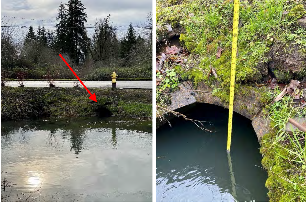
Figure 2. Validation measurement location (48-in. culvert underneath Ridder Road)
