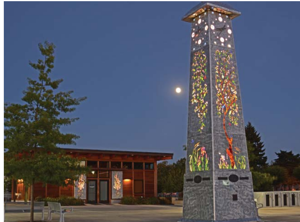
The metal and glass “Clock Tower” sculpture by Jerry Werner located at the Wilsonville Transit Center also contains video cameras and public address system. Credit: City of Wilsonville.
