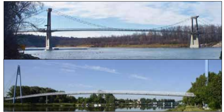
Community members may weigh in with their preference for a suspension bridge (top) or cable stay bridge (bottom), two bridge types advanced by the French Prairie Bridge Task Force and City Council for further consideration.
