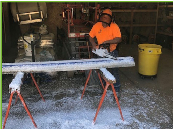
Shaving off two inches from wheel stop
