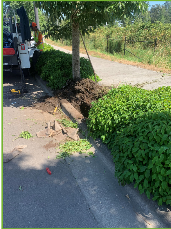
Digging up irrigation
