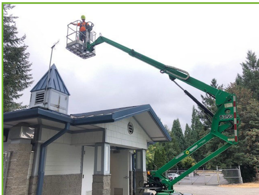
Pump station antenna replacement
