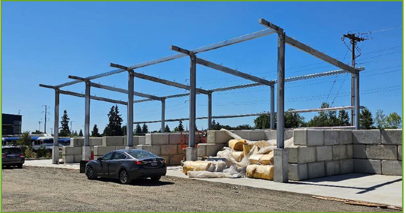
Material storage bins (building E)
