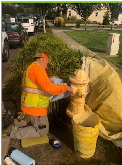
Prepping to paint
