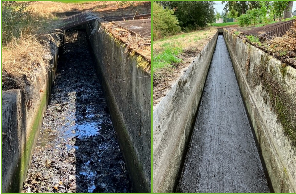
Stormwater level spreader—Before and After
