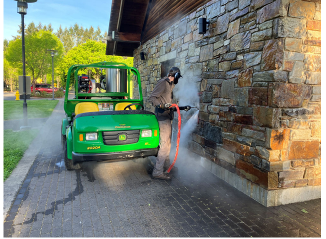
Building Clean Up
