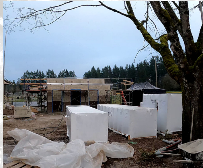
Building Is Roof Ready
