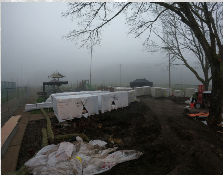
CMU Block Onsite
