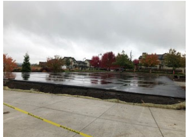
Tennis Court Construction
