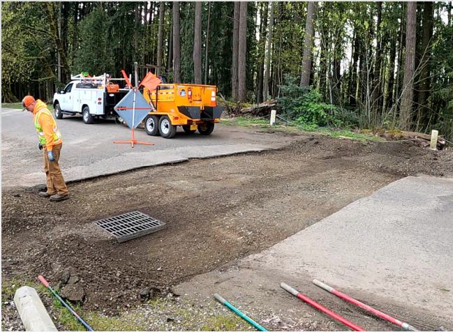
Preparing Base Gravel
