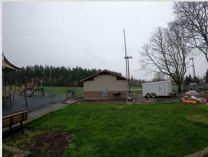
Plumbing Contractor Onsite
