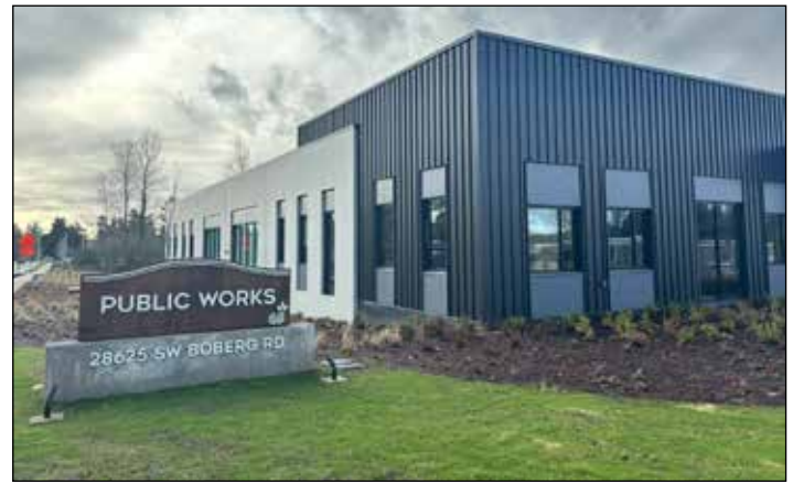
The City’s new Public Works Complex on Boberg Rd. centralizes maintenance activities and provides a seismic-resilient emergency operations center.
