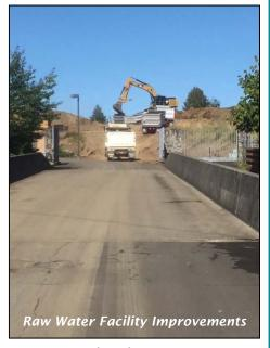
• Raw Water Facility Improvements This capital improvement project is under the management of the Willamette Water Supply Commission and the Tualatin Valley Water District. Improvements include seismic upgrades to the existing intake facility and river embankment, as well as the installation of a 66" raw water pipe and an 8" domestic City water pipe. The Erosion Control and Public Works Permits have been issued. Construction began in July 2020.
