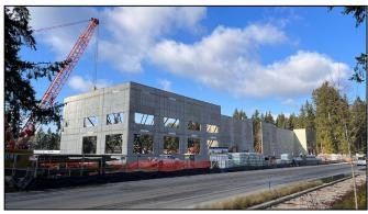
New concrete wall panels being installed at the Grahams Ferry Industrial Center on Garden Acres Road
