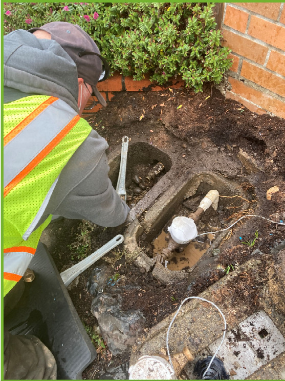
Steve Gering fixing a domestic meter
