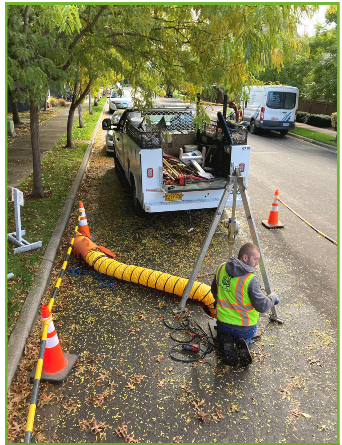
The orange tube circulates air in the manhole
