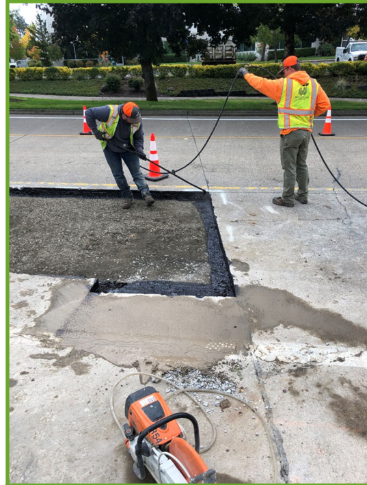
Sealing around the new section
