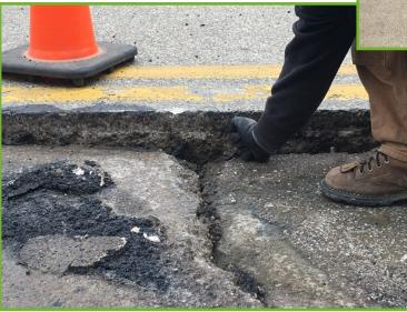
The mastic covering will provide a smoother driving surface and a more permanent solution. Additionally, crack sealing was applied to the concrete panel to prevent any extra water from getting in to the subgrade and eroding away the base rock.
