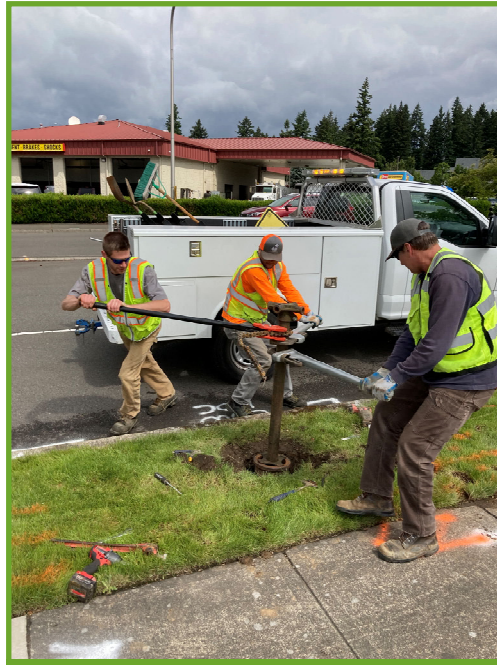
Replacing stem
