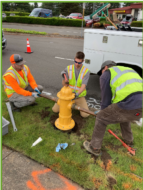
Setting new hydrant
