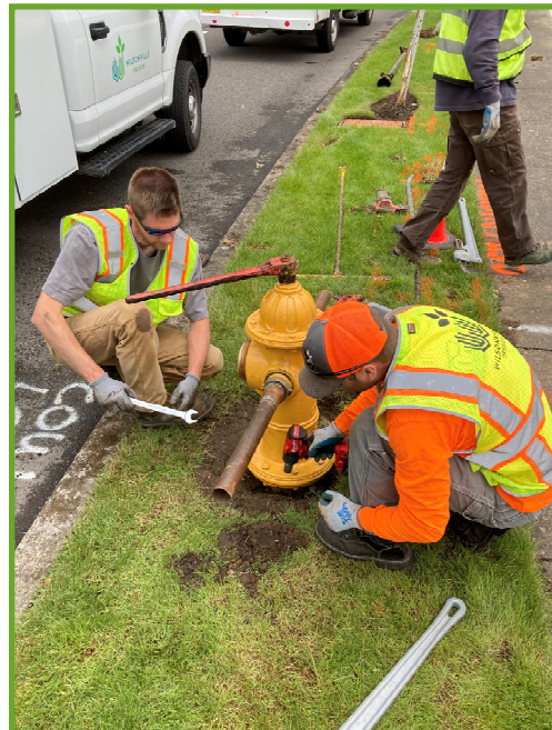
Securing the new hydrant
