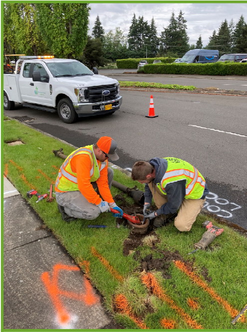
Removing inner stem
