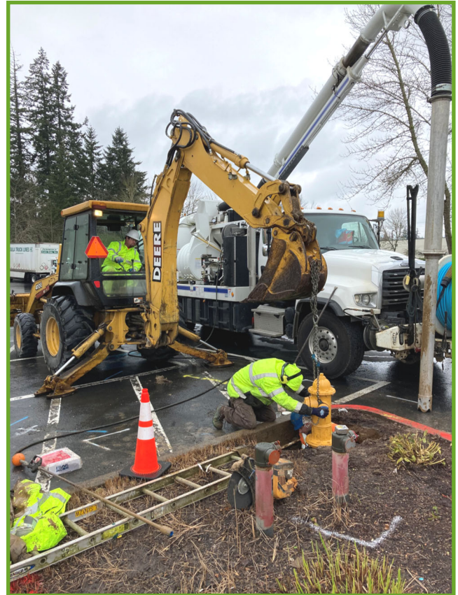
Installing a new hydrant
