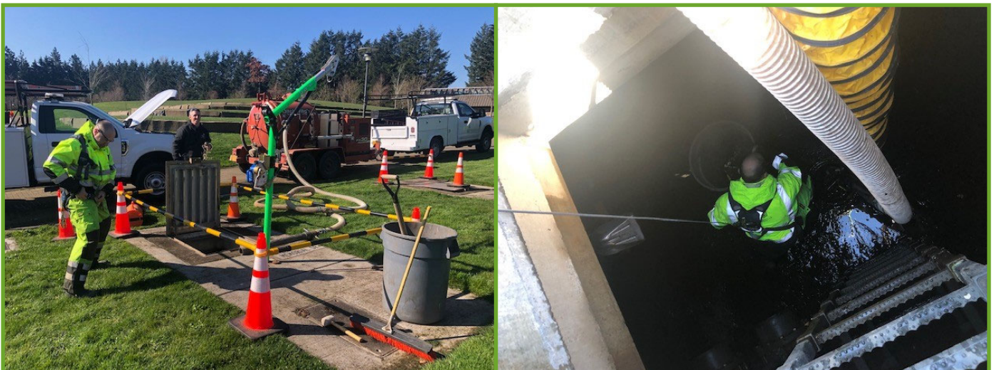
Preparation and entering an underground confined space
