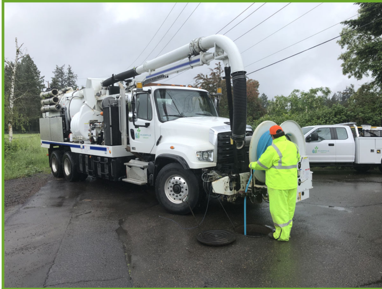
Flushing the sewer line
