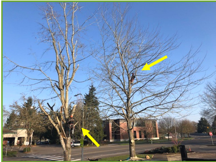
Contractors set the rigging
