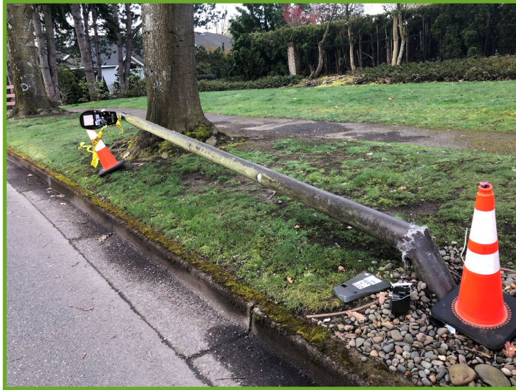
Damaged light pole
