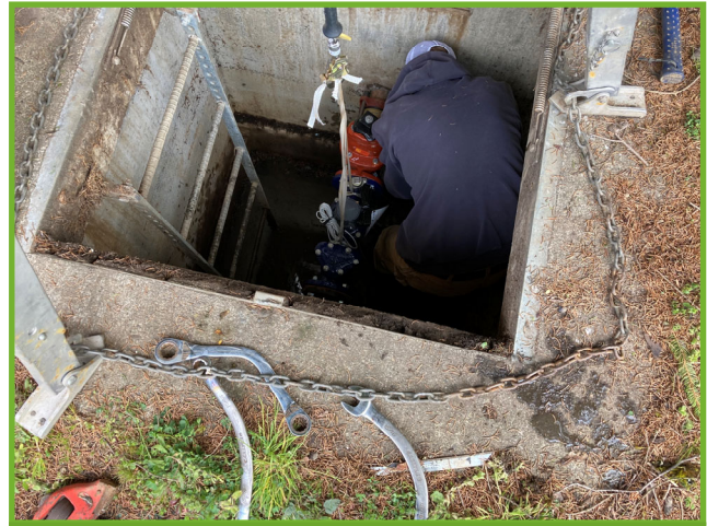
Sam performs a meter replacement
