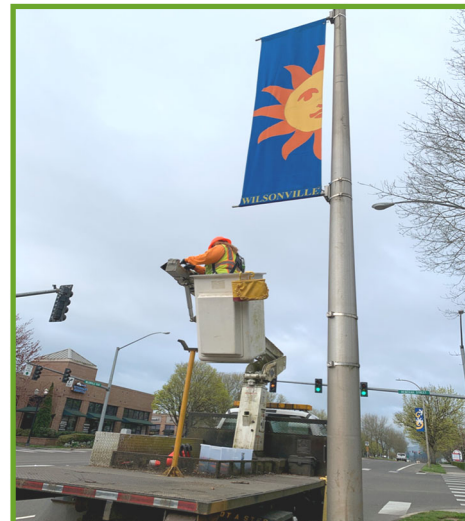
Coming down in the bucket lift
