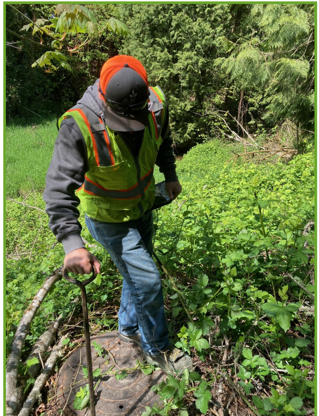
Randy lifting a manhole lid
