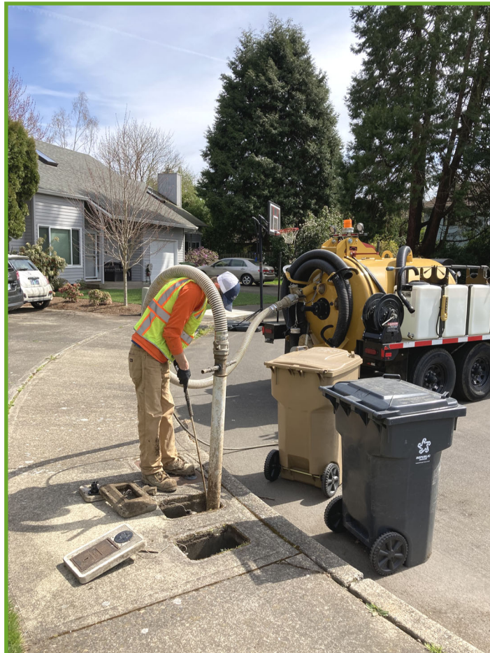
Sam cleaning out meter boxes
