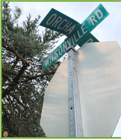
Bent street sign
