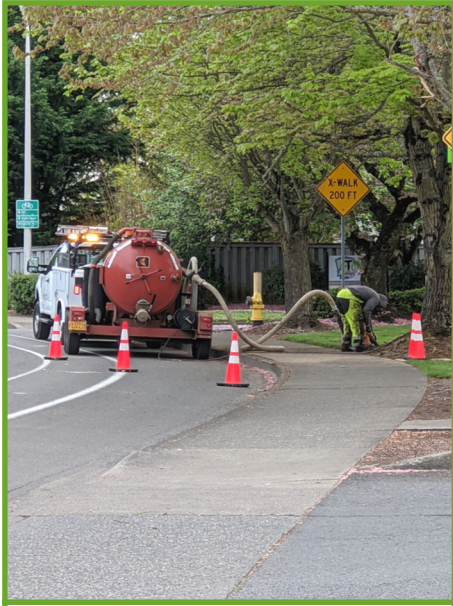
Operating the Ditch Witch
