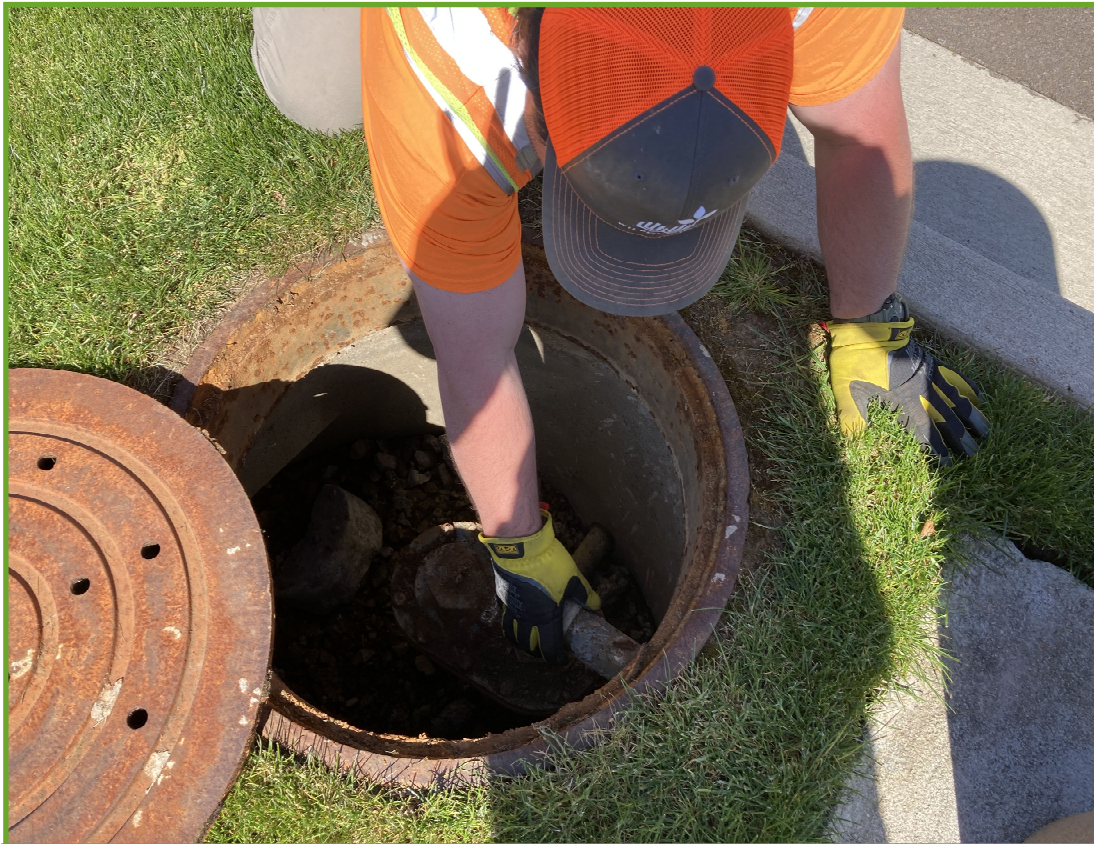
Chad inspecting an Air Release Valve (ARV)
