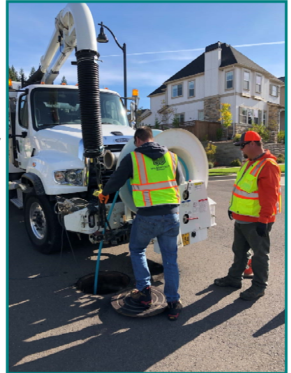
Kyle Bean and Chad Whiting Cleaning the Sewer
